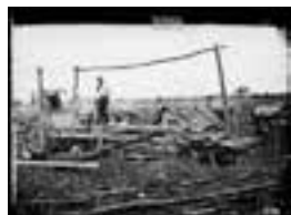
Pitsawing timber, Gulgong 1872 a2822085
